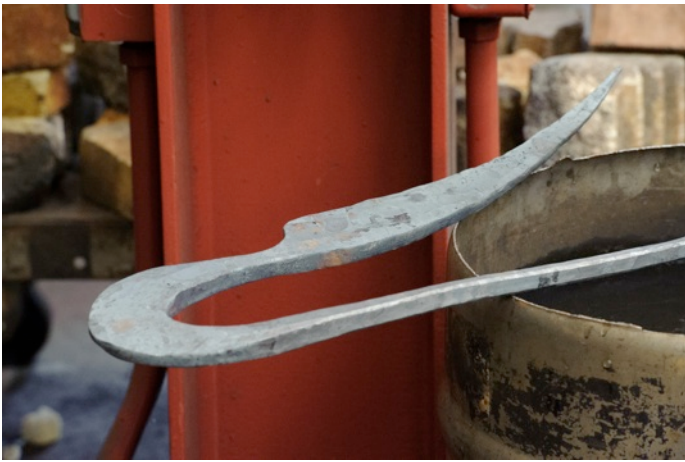
Core element ready for the final bending
